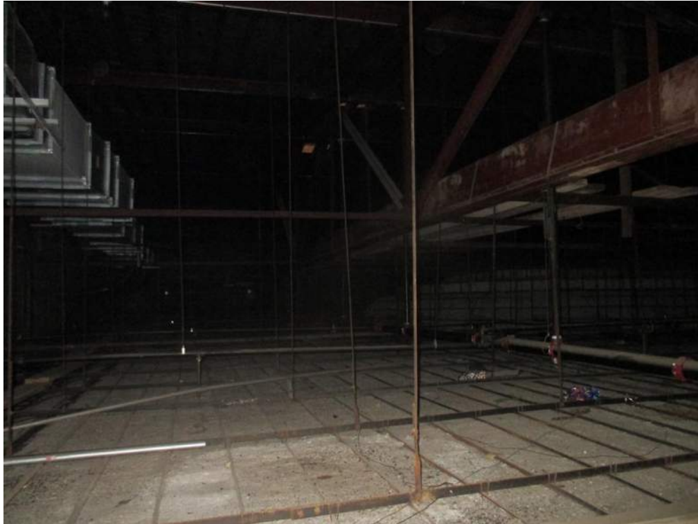
Photo 3 General view of suspended ceiling support system
