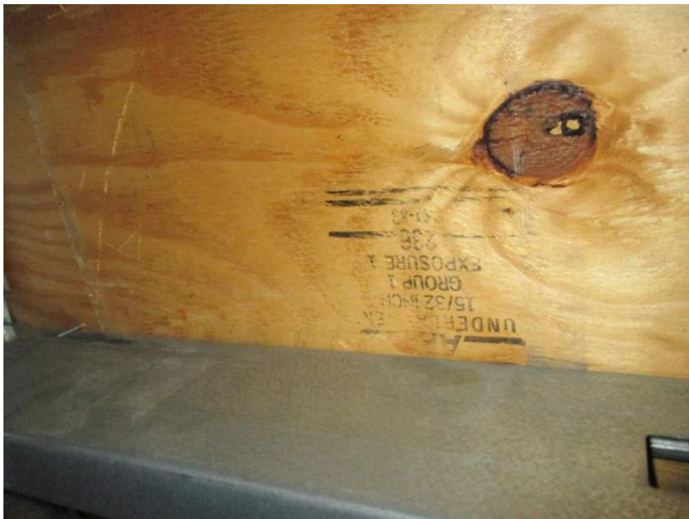
Photo 19 Underside of floor decking for Black Box Stage
