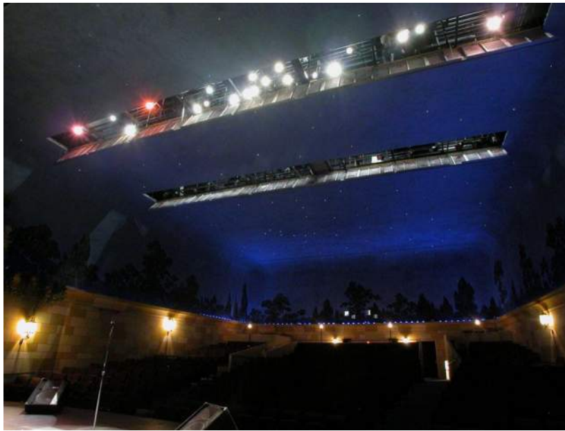
Fig. 3 In this example of modern technology incorporated in the "plaster on expanded metal lath" ceiling of an atmospheric cinema/live theatre, when not in use as a theatre its lighting can be closed off behind a system of numerically controlled doors that when closed leave a smooth ceiling for the projection of cloud effects typical of an atmospheric cinema.
