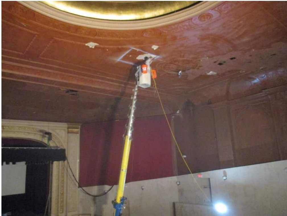
Photo 1 Plaster ceiling being cut to permit evaluation
