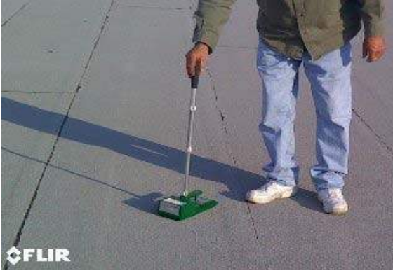
PHOTO 1 Lower Roof Section: Tramex meter was place on roof surface every 2-4 feet in grid pattern.
