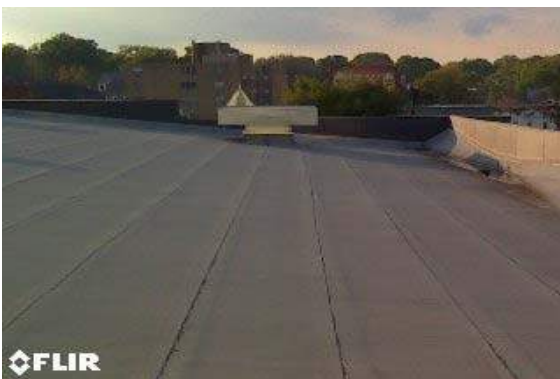
PHOTO 5 Lower Roof Section: Lower roof appears to be in excellent condition.
