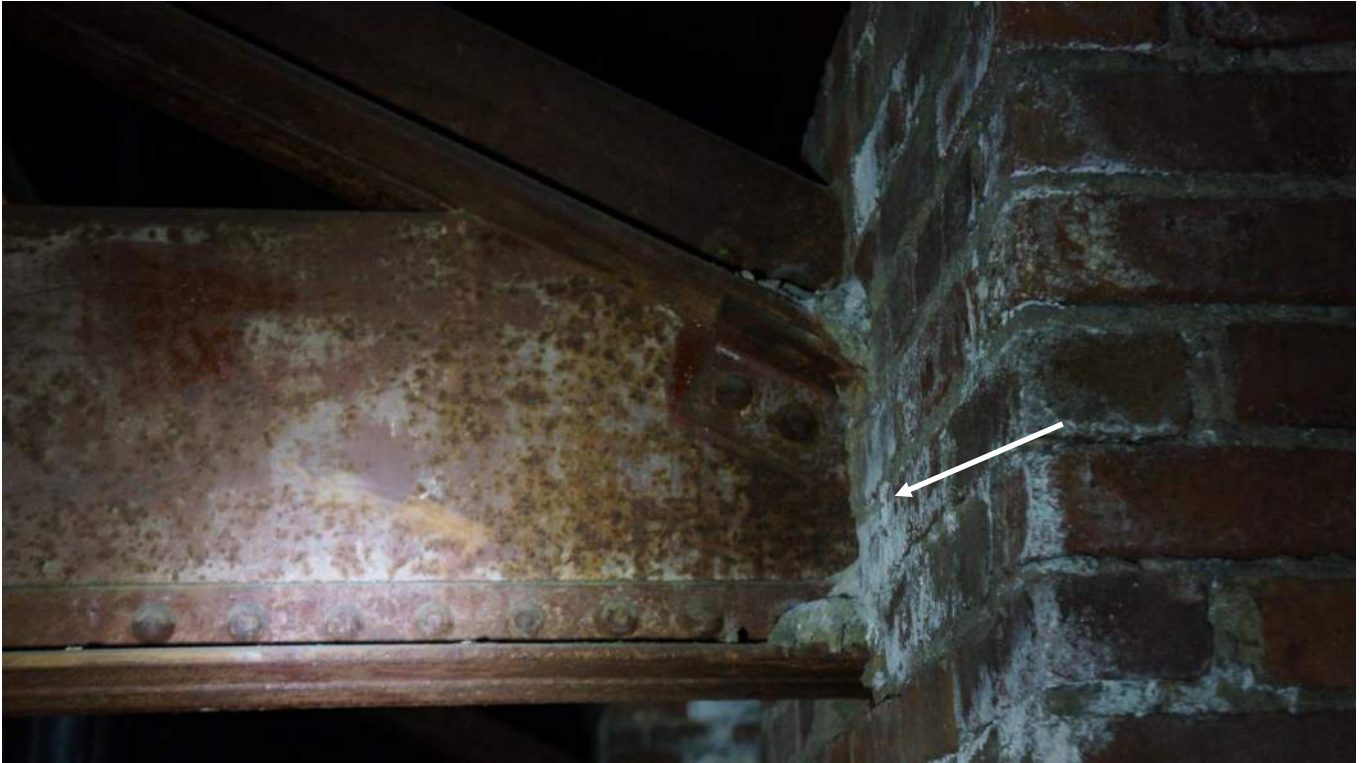
Photo 9 Masonry bearing of the roof truss
