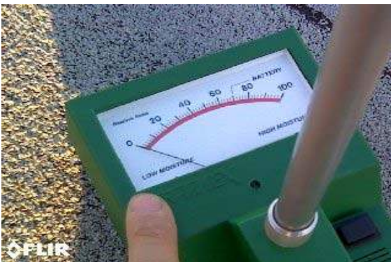
PHOTO 11 Upper Roof Section: Zero moisture detected throughout roof area.
