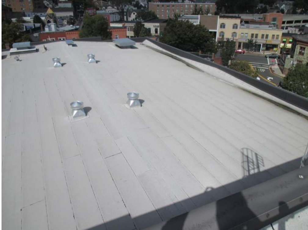
Photo 5 General view of theatre roof
