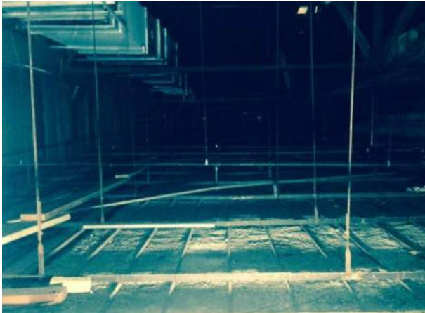
Fig. 1 Typical view across the plenum indicates a systematic and orderly layout. Attached to the plaster by wires, the typical Chicago Bar system is spaced at 16: with the opposing angle irons at 5' centers. Verticals bolted to these are 1" X 1/8" straps.
