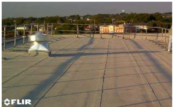
PHOTO 12 UPPER Roof Section: Upper roof appears to be in excellent condition.
