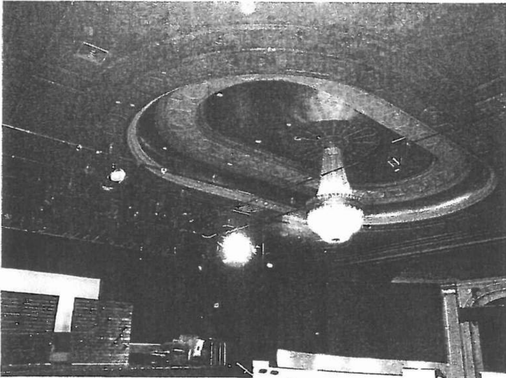
Photo 13 View of the plaster ceiling over main seating area.
