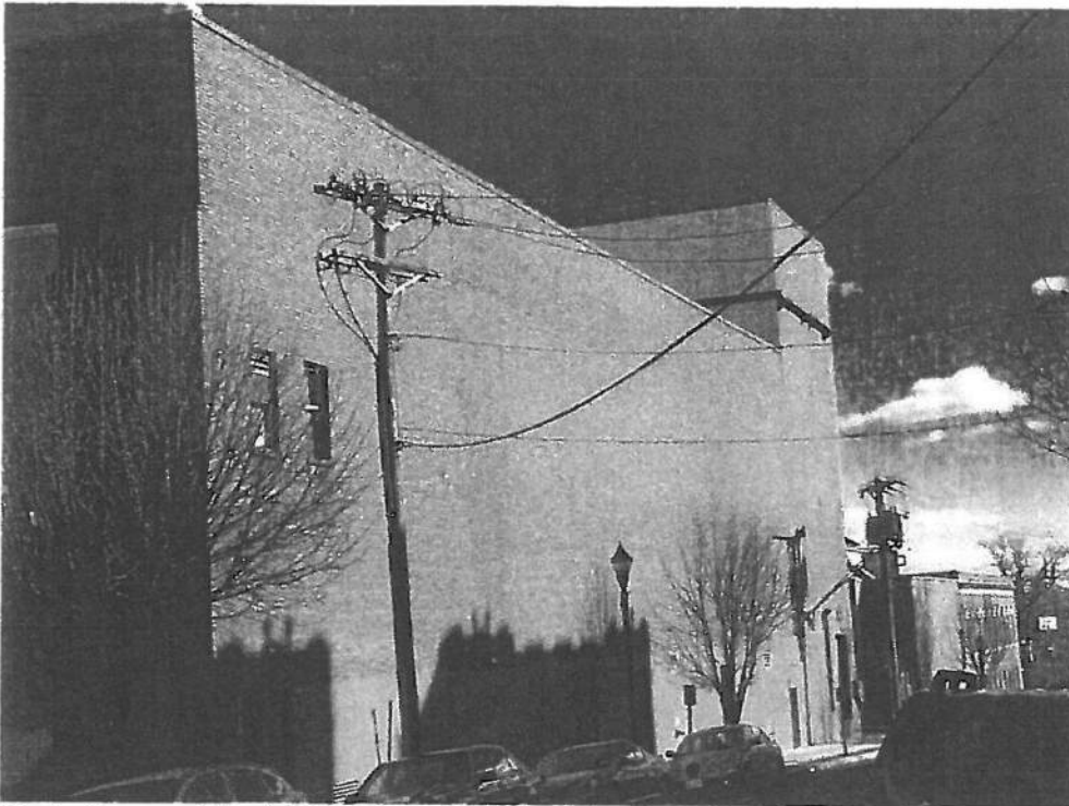
Photo 3 South Elevation of original theater building (viewed from Sylvan Street)
