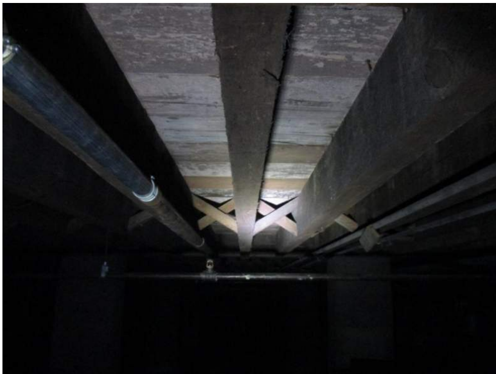
Photo 17 Floor joists under proscenium stage
