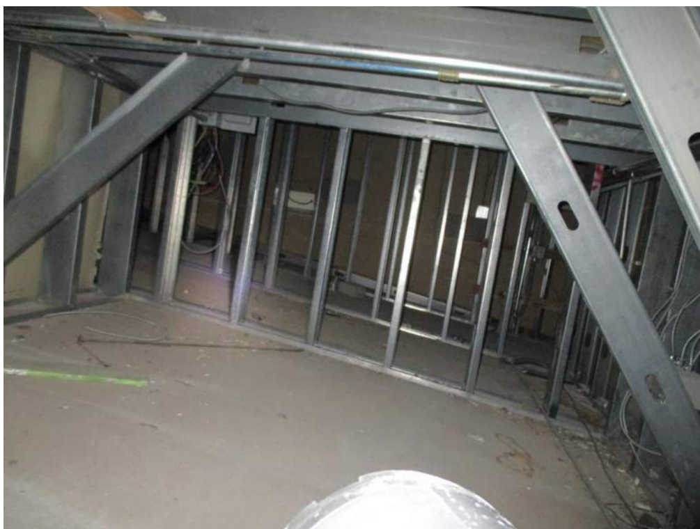
Photo 20 Cold formed steel joists under black box stage
