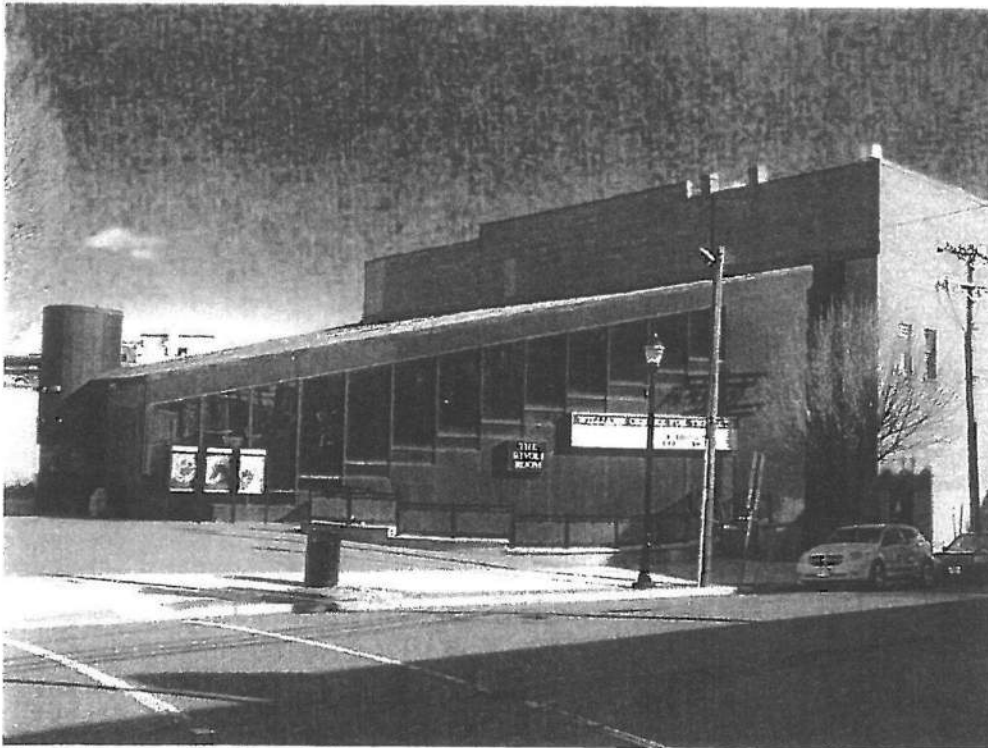
Photo 4 1980's addition to original theater building (viewed from Sylvan Street). Note the original facade and marquee was removed to make this addition.
