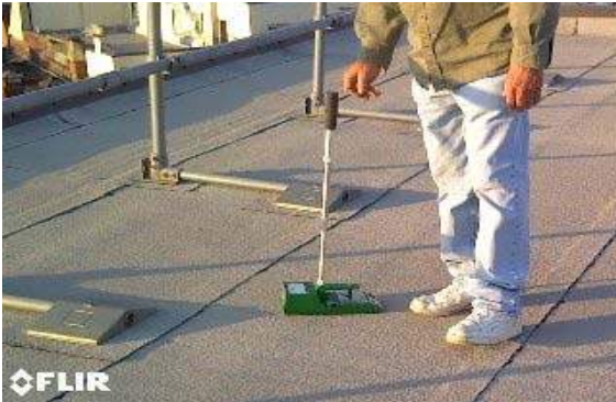
PHOTO 9 Upper Roof Section: Tramex meter was place on roof surface every 2-4 feet in grid pattern.
