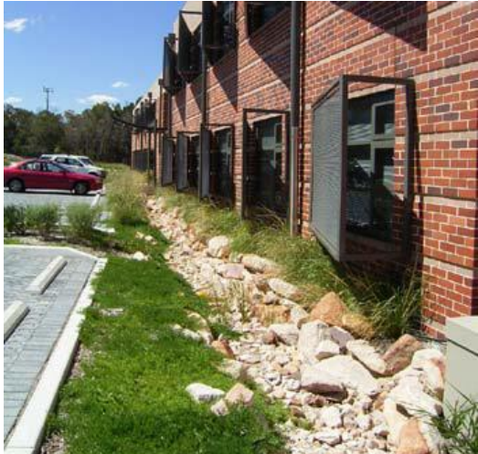
Permeable parking lot and bioretention system for commercial buildings
