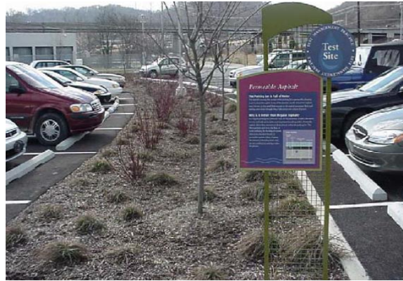
Bioretention swale in a parking area
