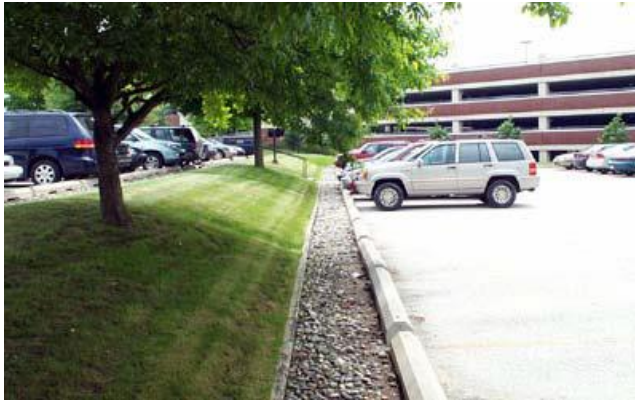
Infiltration beds in a parking lot
