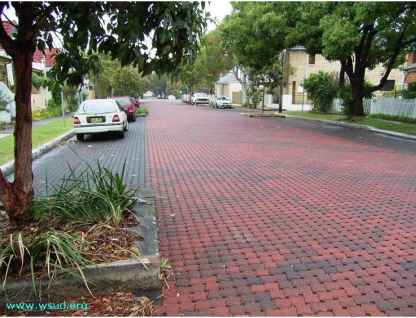
Permeable paver retro-fit for a residential street
