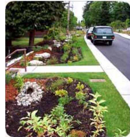
Bioswale along a Residential Street
