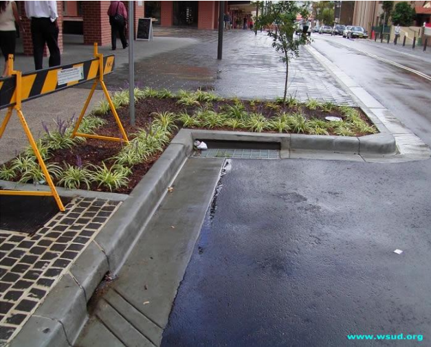
Street tree stormwater treatment retro-fit
