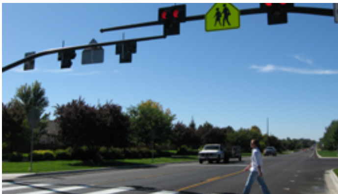
Figure 10. HAWK beacon (Courtesy of BPRC).
