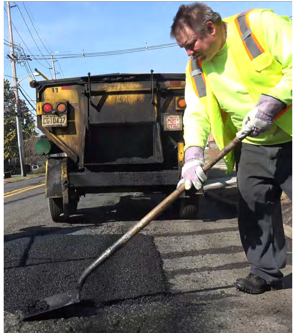
Road Repair. Source: Donna Brennan, Bergen County
