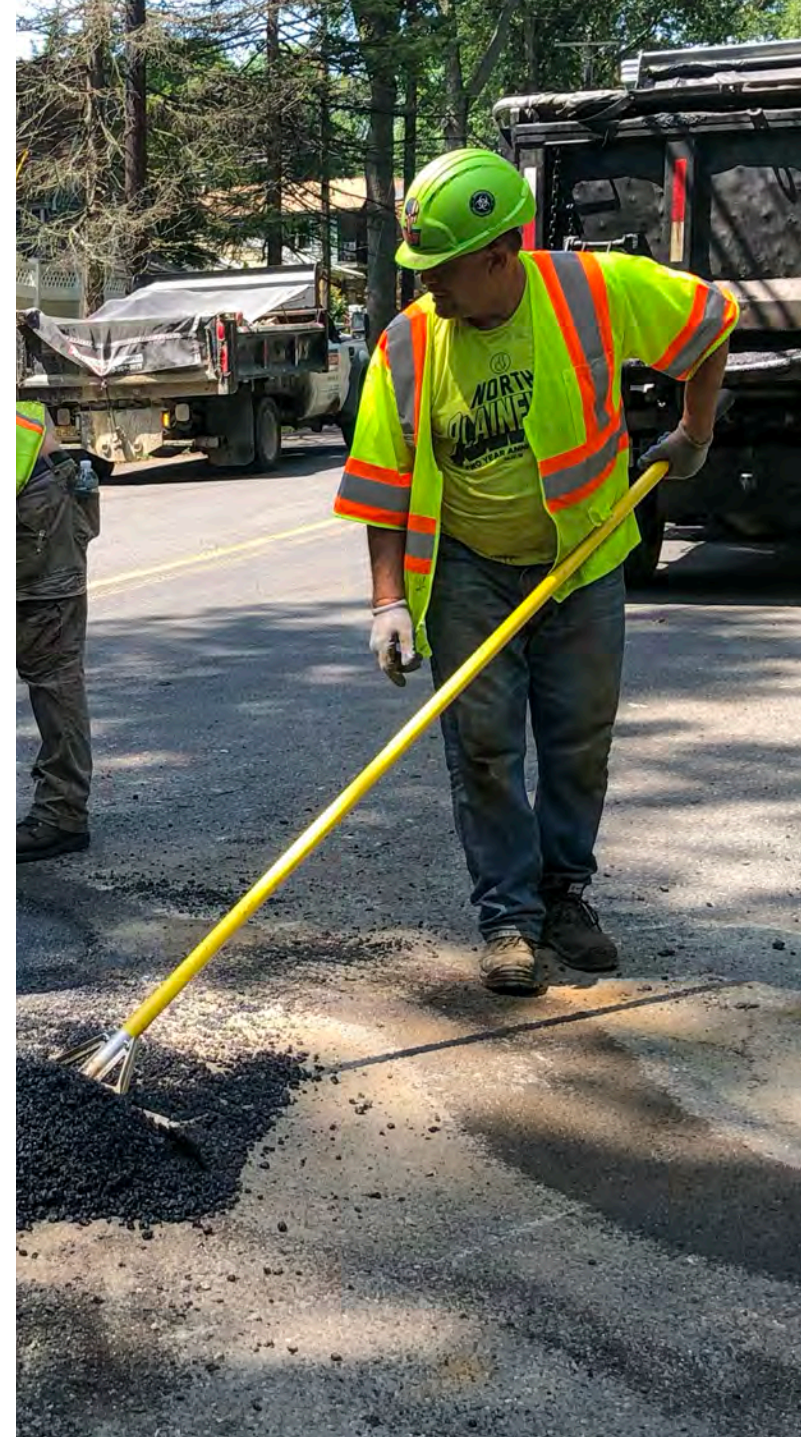
Road Repair. Source: Donna Brennan, Bergen County
