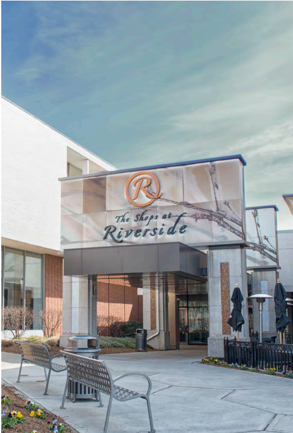
The Shops at Riverside. Source: Donna Brennan, Bergen County
